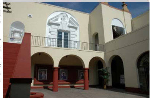
The Courtyard lobby after a little sprucing up offers a glimpse of how extraordinary the Fox Theater will be when the six phase restoration is complete.
